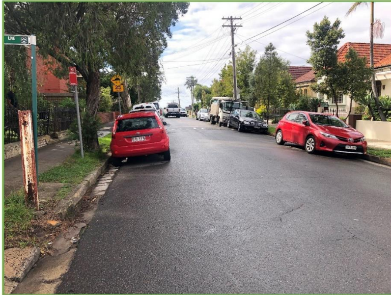
View east along Warren Road from Stinson Lane
