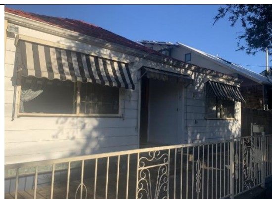
Figure 2: Site photo prior to demolition.
