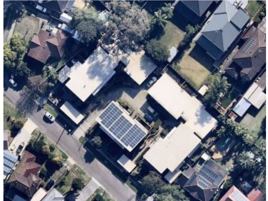
25kW solar system sharing into apartments.
