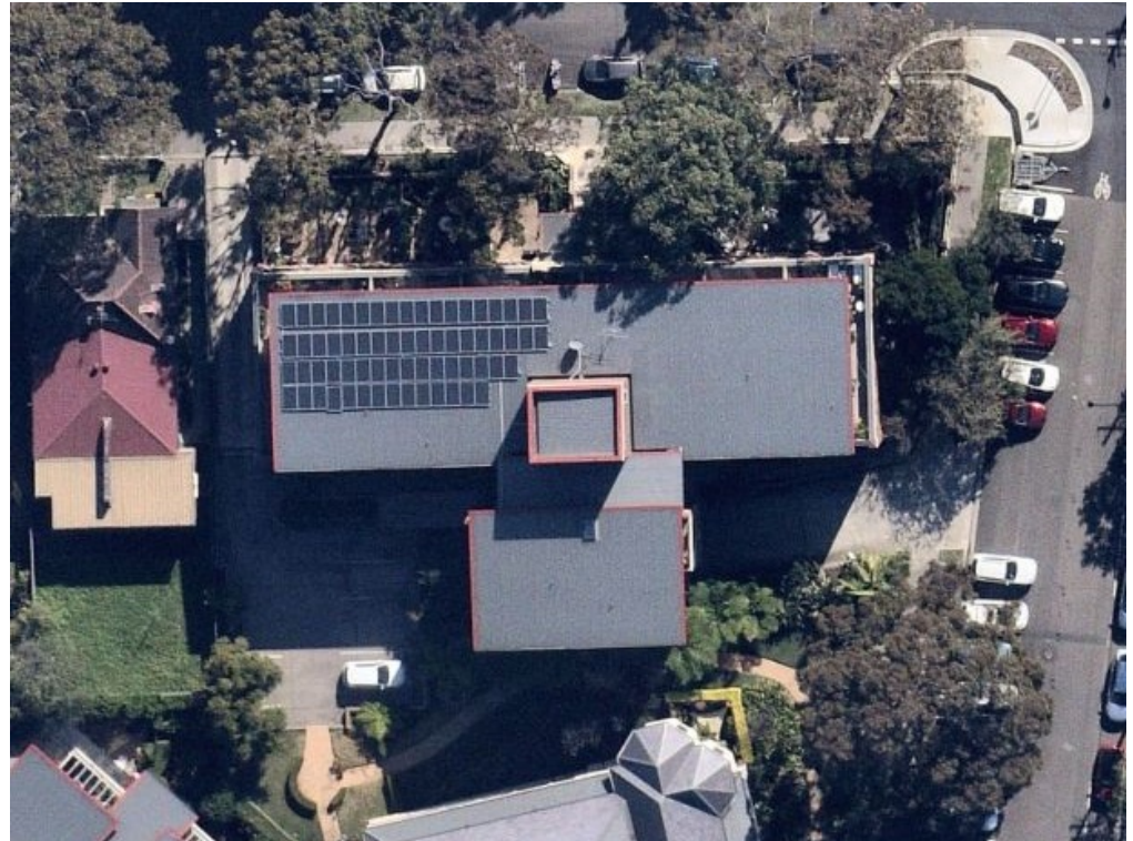
80A Victoria Rd Marrickville. ~20kW solar system on apartment block
