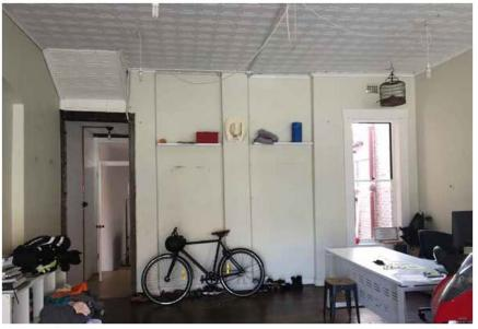
**Figure 19** The rear of the shop. Apart from the pressed metal ceiling the fabric is extensively altered. The window is aluminium framed.
