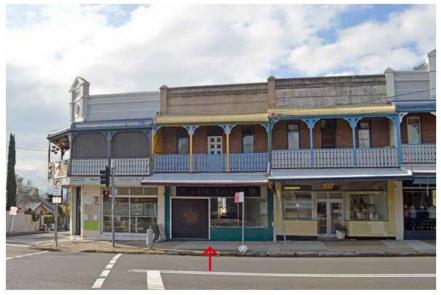
Figure 6 The Catherine Street elevation. The shopfront has an intrusive roller shutter. The balcony, the rendered parapet and first floor openings are mostly original.
