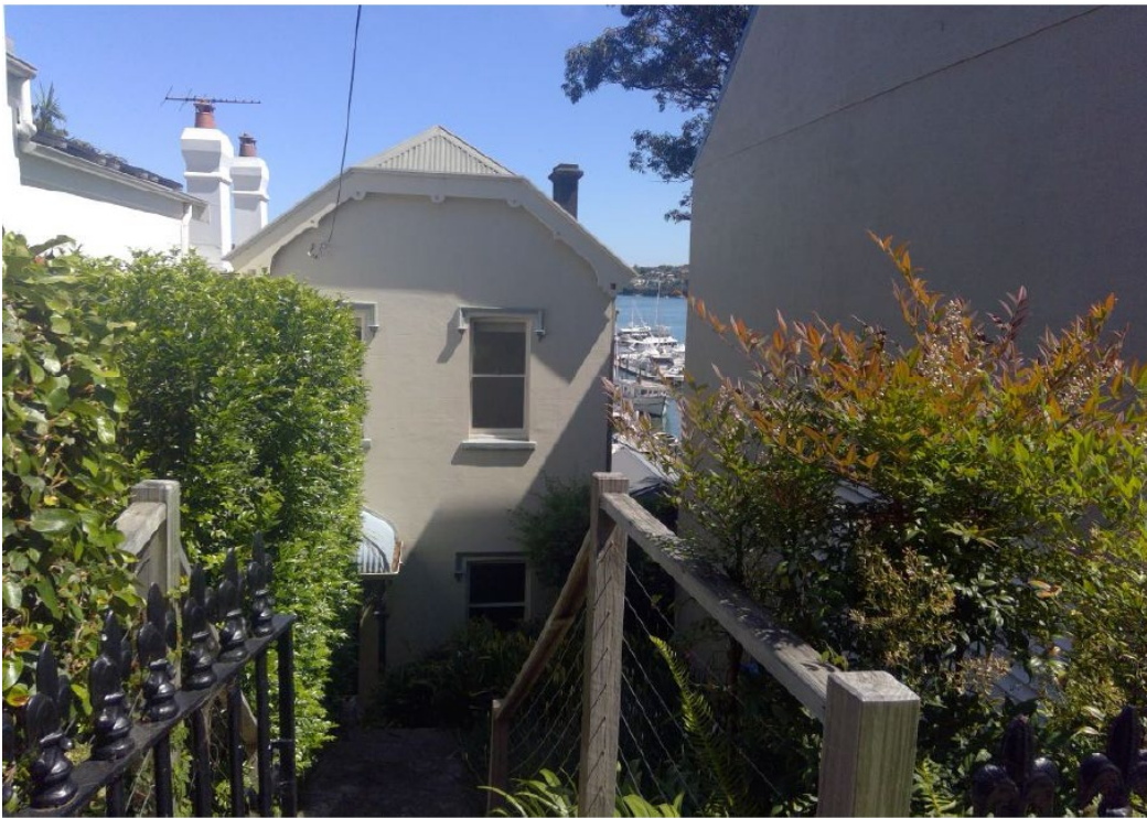
View on footpath in front of front gate of No.9 Phoebe
