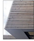
(G) HARDWOOD TIMBER CLADDING
