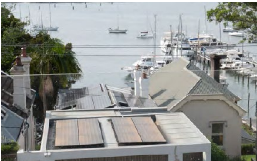
Image showing location of solar panels on the roof of 11 Phoebe with the existing dwelling at 9 Phoebe in the background.
