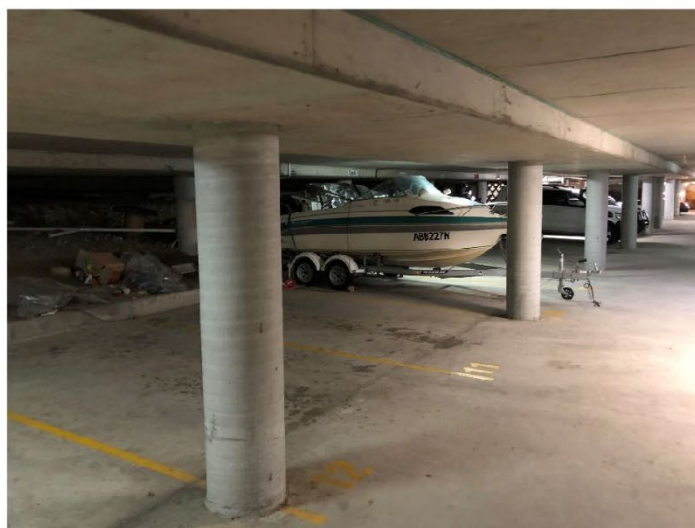
Figure D: Underground Level Parking within 111 Moore Street
