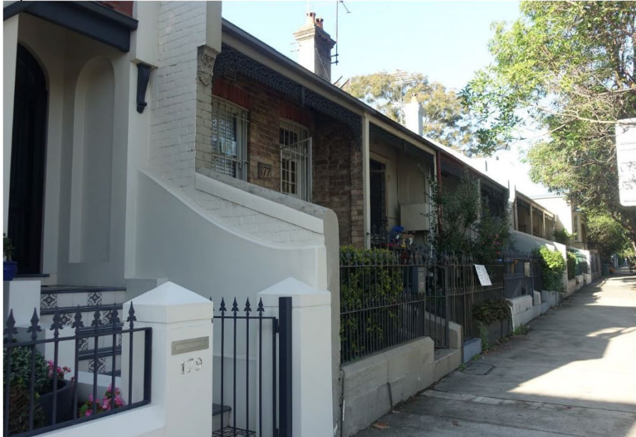
Front view of the row Nos 177 to the left end adjoining No 175, then 173, 171, then a gap given access to the rear, then a further row of three, Nos 169, 167 & 165. They were evidently built by the same hand.
