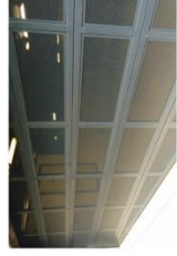
RS - CAR PARK ENTRY DOOR
