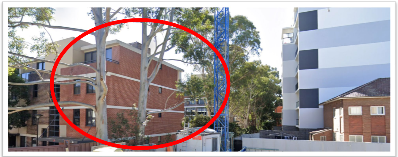
Figure 2 – Window openings of 1 Brown Street facing 6 Murrell Street in red circle.
