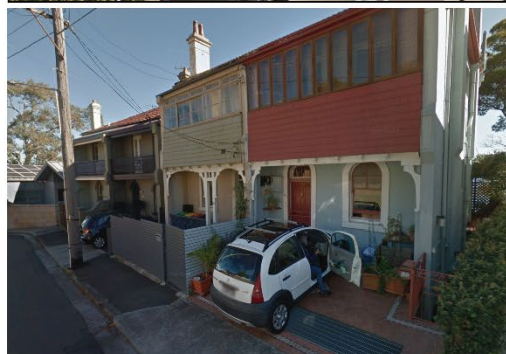
Figure 17: No. 60 and No. 56 Louisa Road are Victorian era terraces with carparking spaces.
