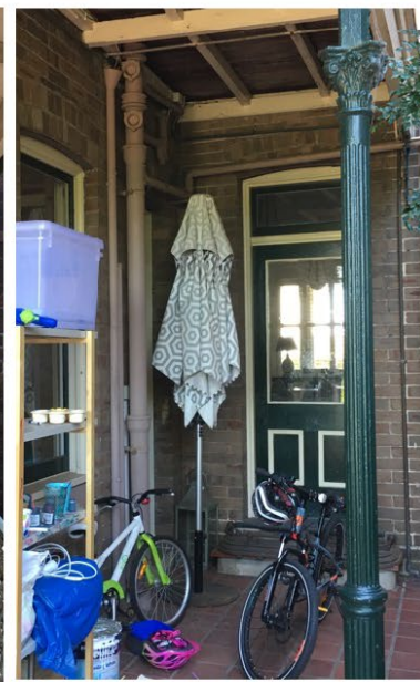
Figure 10: The Ground Floor underneath the timber verandah.
