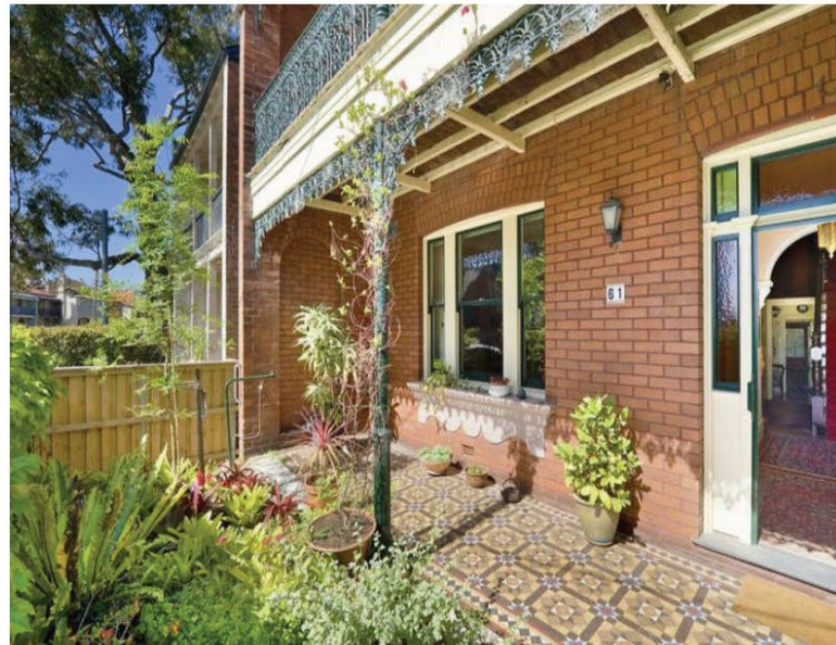
Figure 7: The front verandah with encaustic tile flooring.
