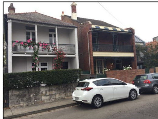
Figure 18: No. 63 Louisa Road to the North.
