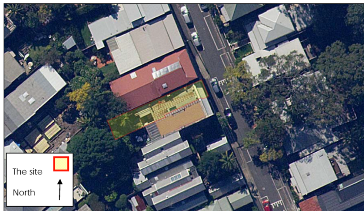
Figure 1: Aerial view of the site in its immediate context (© six viewer)
