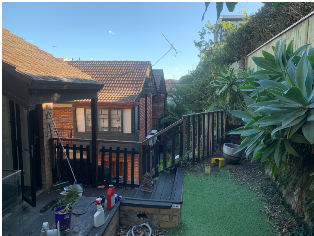
Existing rear private open space – comprised of decking, paved area and void between building and escarpment
