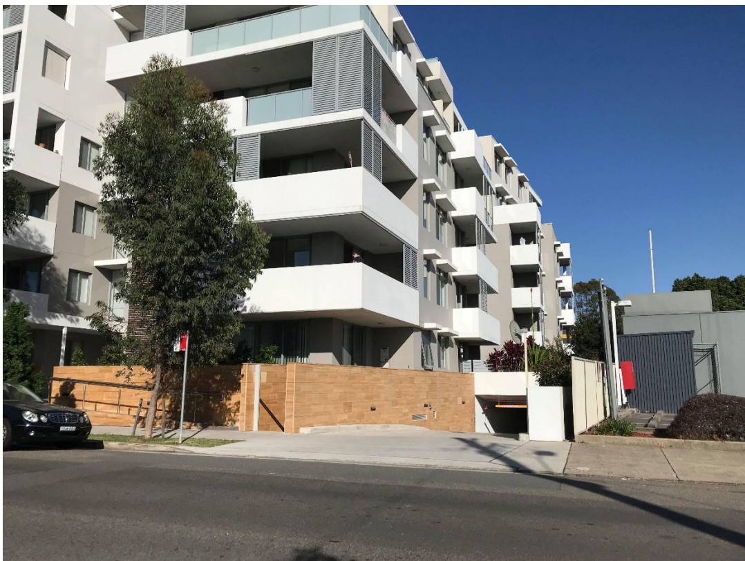
Figure 5: Victoria Street access to basement car park of building at No. 1-7 Victoria Street. The subject proposal relies on this vehicular access through this entrance which has a right-of-way.
