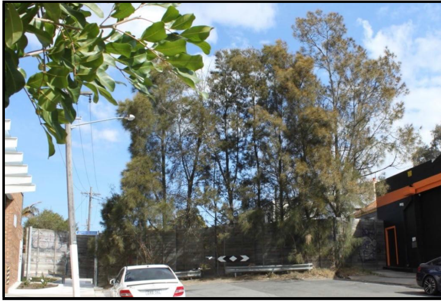
Figure 8: Cul-de-sac and dividing wall in Lonsdale Street with the subject site to the right
