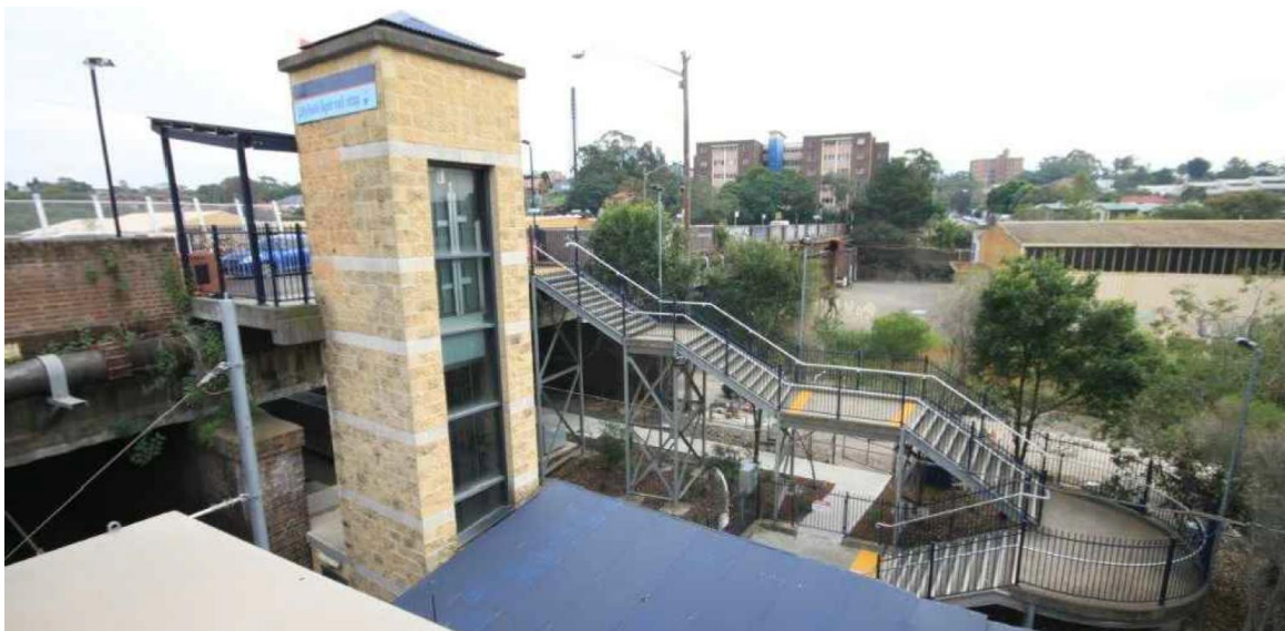
Figure 3: Photo of Lilyfield Light Rail Station
