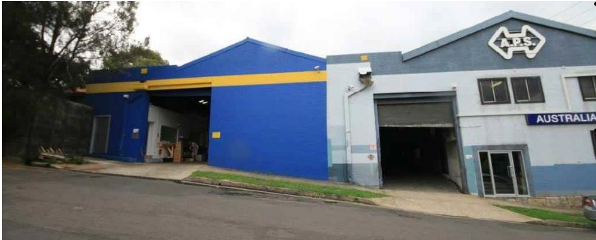
Figure 7: Photo of 36 Lonsdale Street, Lilyfield
