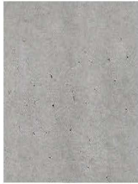
CONC01 OFF FORM CONCRETE
