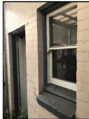
Figure 31. View to rear of building.
