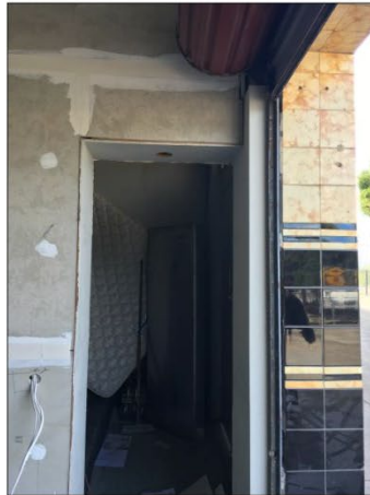
Figure 24: Detail of the access to the under-stair storage area.
