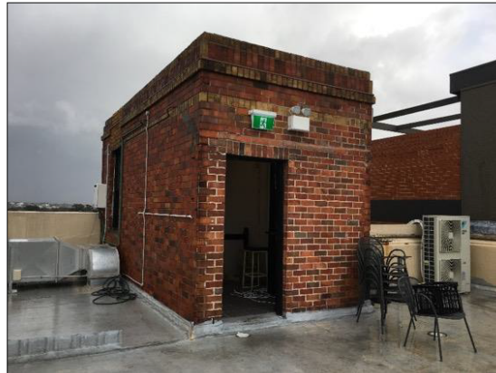
Figure 19: Brick fire stair enclosure.
