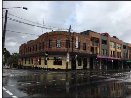
Figure 30: View of the subject site from the east.
