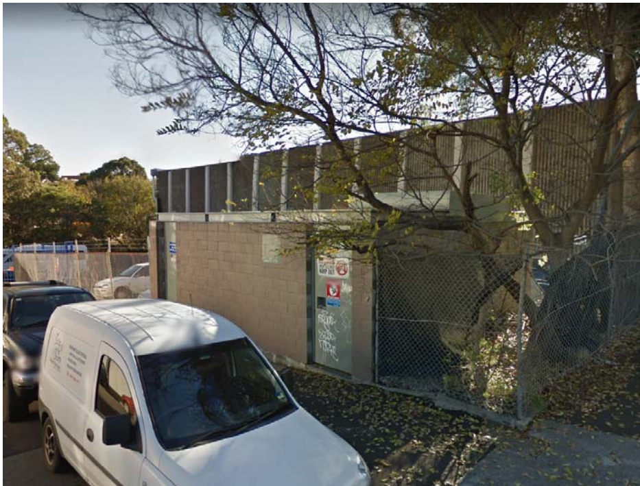
Figure 7 - Kennards Storage Warehouse at 1 - 19 Booth Street opposite the subject site
