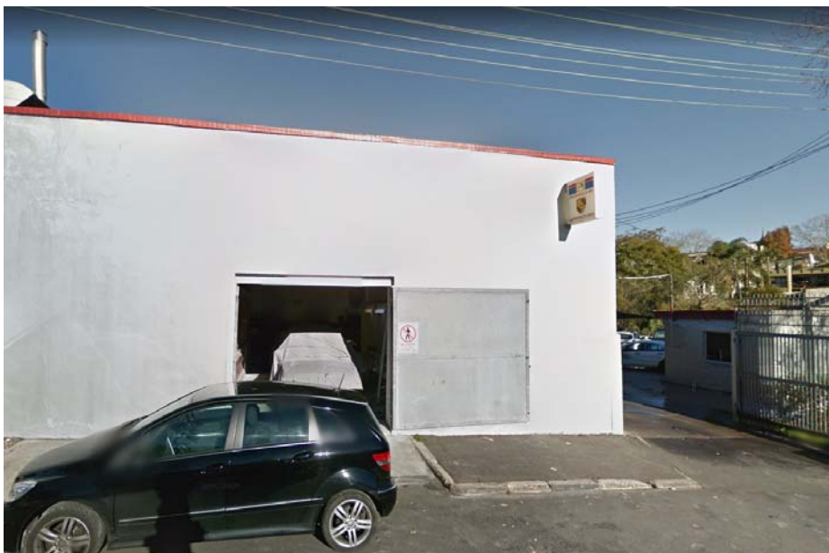
Figure 4 - Existing warehouse when viewed from Chester Street.
