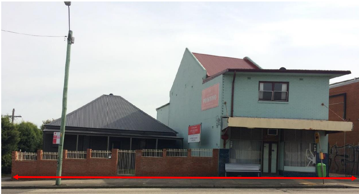
Figure 1: Site viewed from Canterbury Road.
