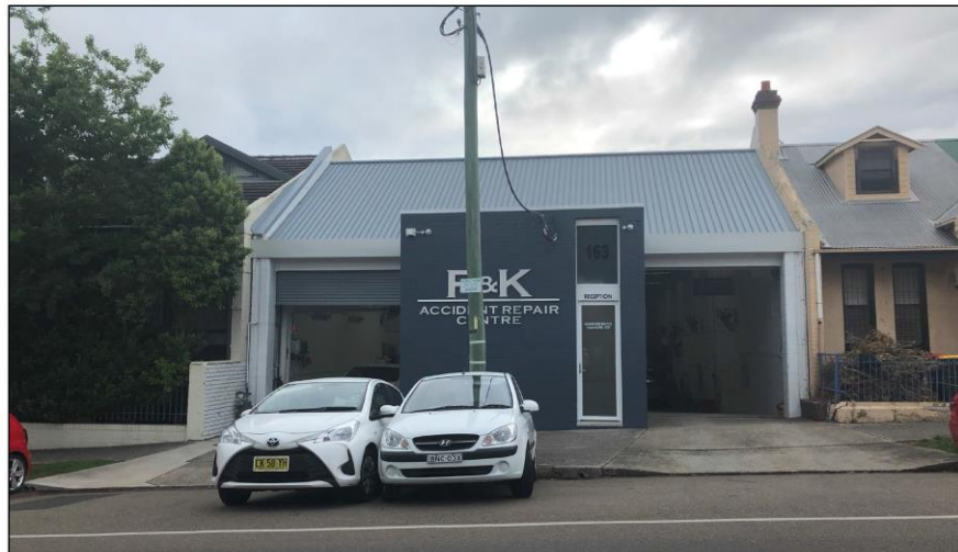
Figure 1: View of the existing development on the site looking east from Catherine Street
