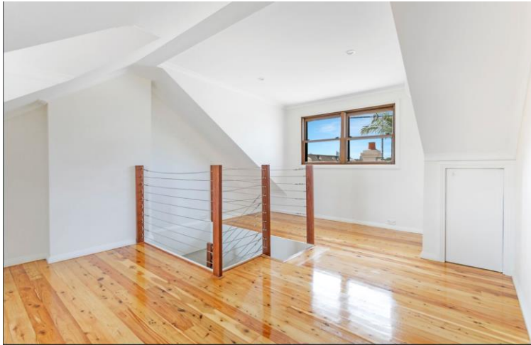
Figure B: View from rear first floor bedroom of No. 161 Catherine Street (b)
