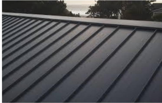
METAL SHEET ROOFING
