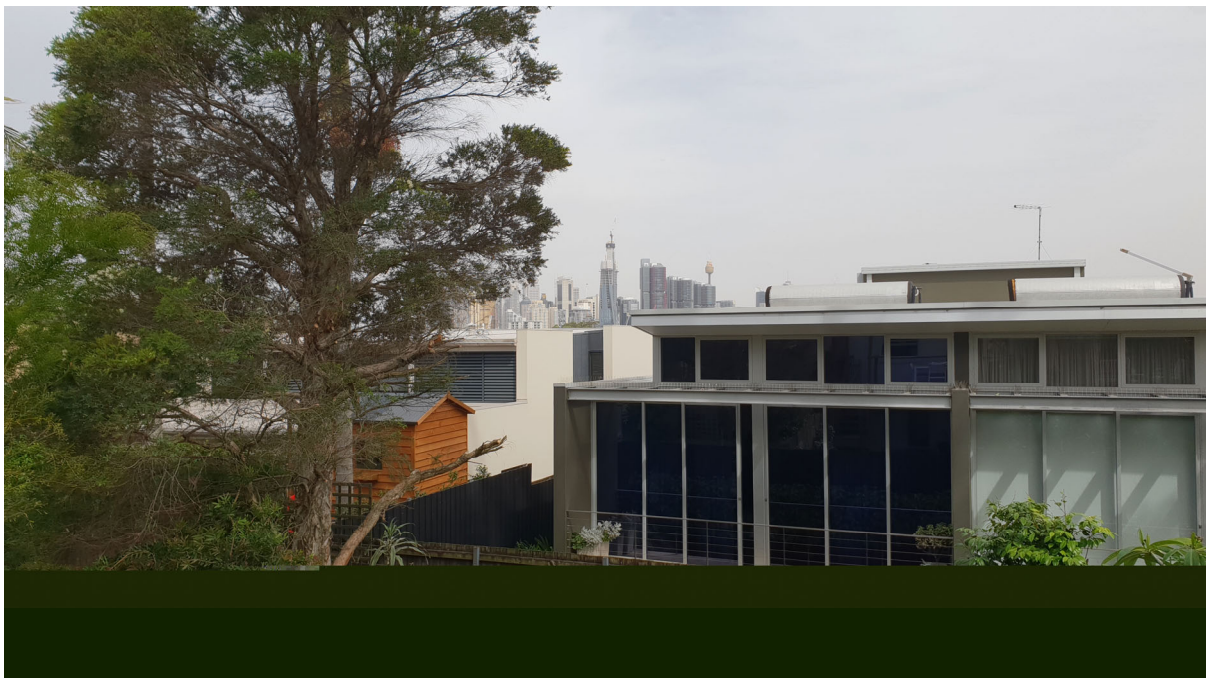
View from elevated ground floor deck
