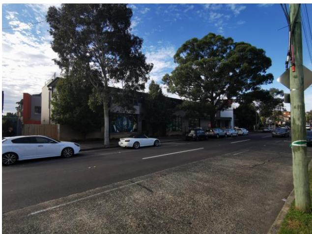
Figure 7 237 Marion Street Development
