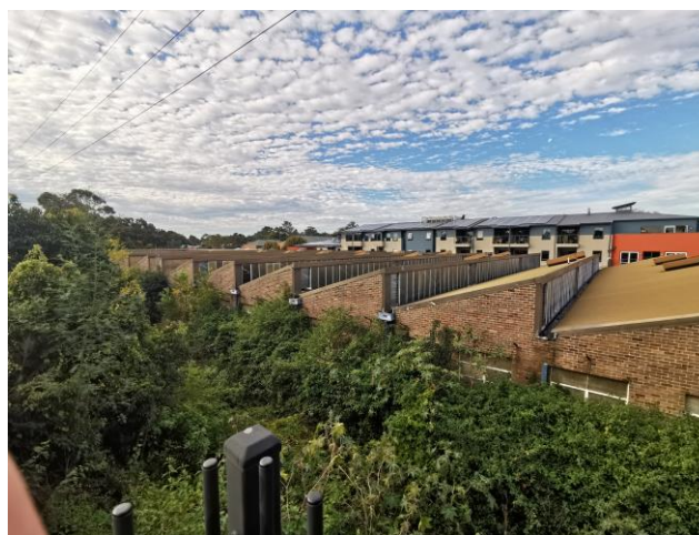
Figure 12 The site, as viewed from Marion light rail stop
