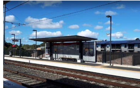
Figure 3.4: Marion Light Rail Station
