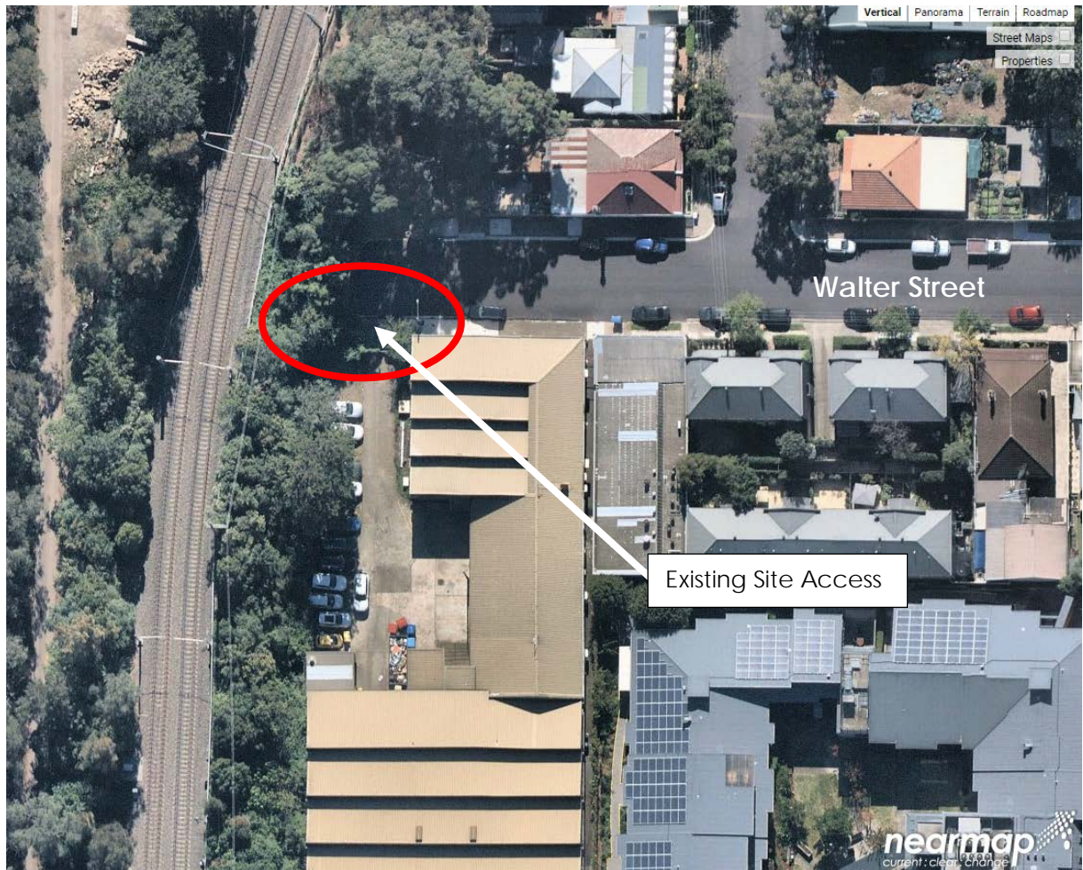
Figure 2.3: Existing Walter Street Site Frontage with Access Driveway
