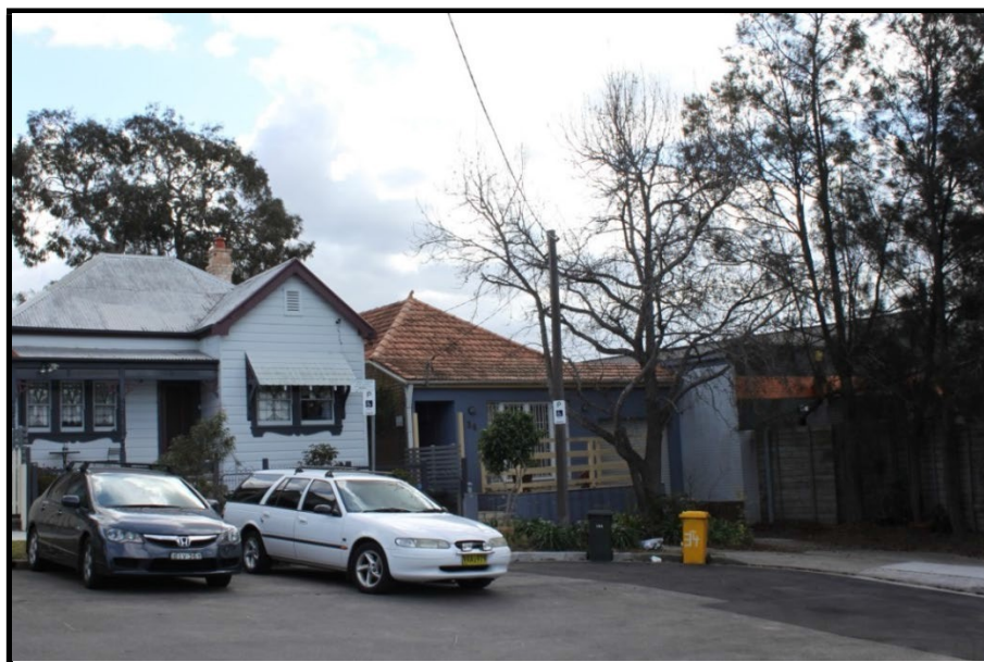
Figure 7: Adjoining Development to the South - 34 & 32 Lonsdale Street
