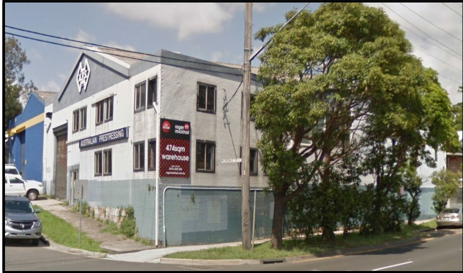
Figure 3: Existing Development on the site - corner of Lonsdale and Brenan Streets
