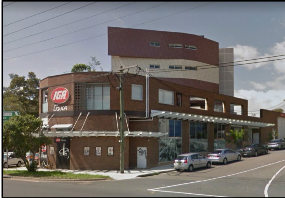
Figure 6: Adjoining Development on the opposite side of Lonsdale Street – IGA site
