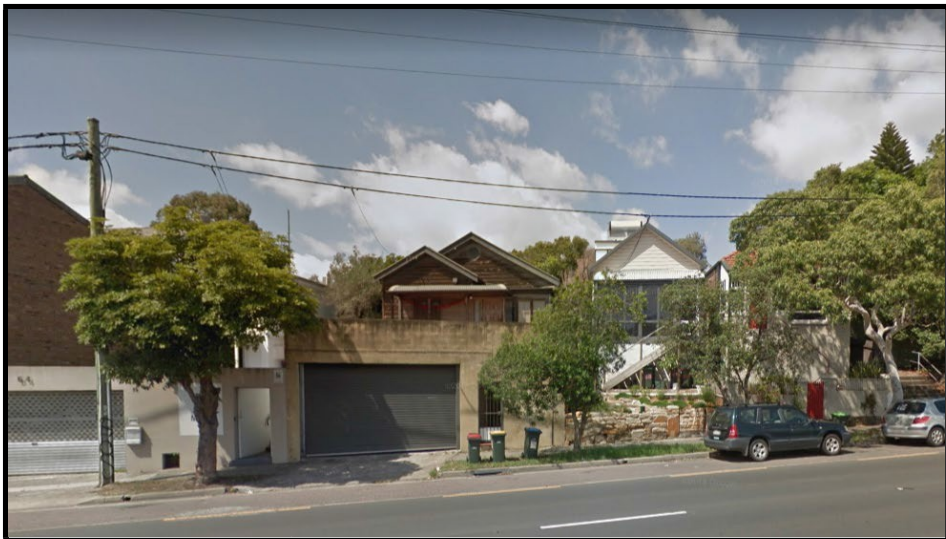
Figure 4: Existing Development on the site - along Brenan Street
