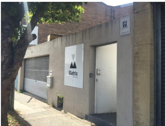
64 Brenan Street (Street frontage)
