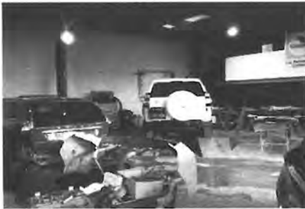
View of 1-5 Chester St, Annandale. Showing Borehole Location BH5 Looking south. Inspected on 13.05.2017
