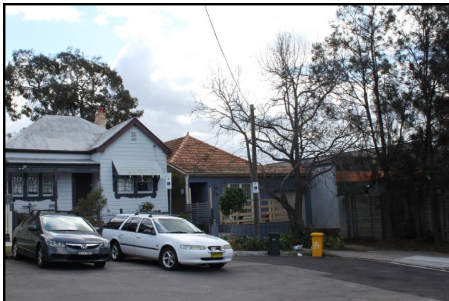
Figure 7: Adjoining Development to the South - 34 & 32 Lonsdale Street
