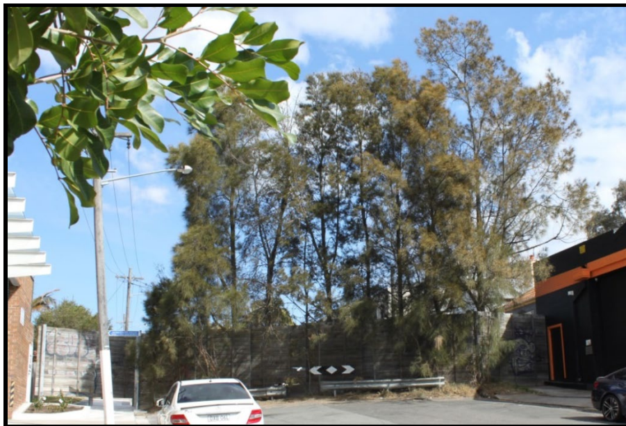
Figure 8: Cul-de-sac and dividing wall in Lonsdale Street with the subject site to the right
