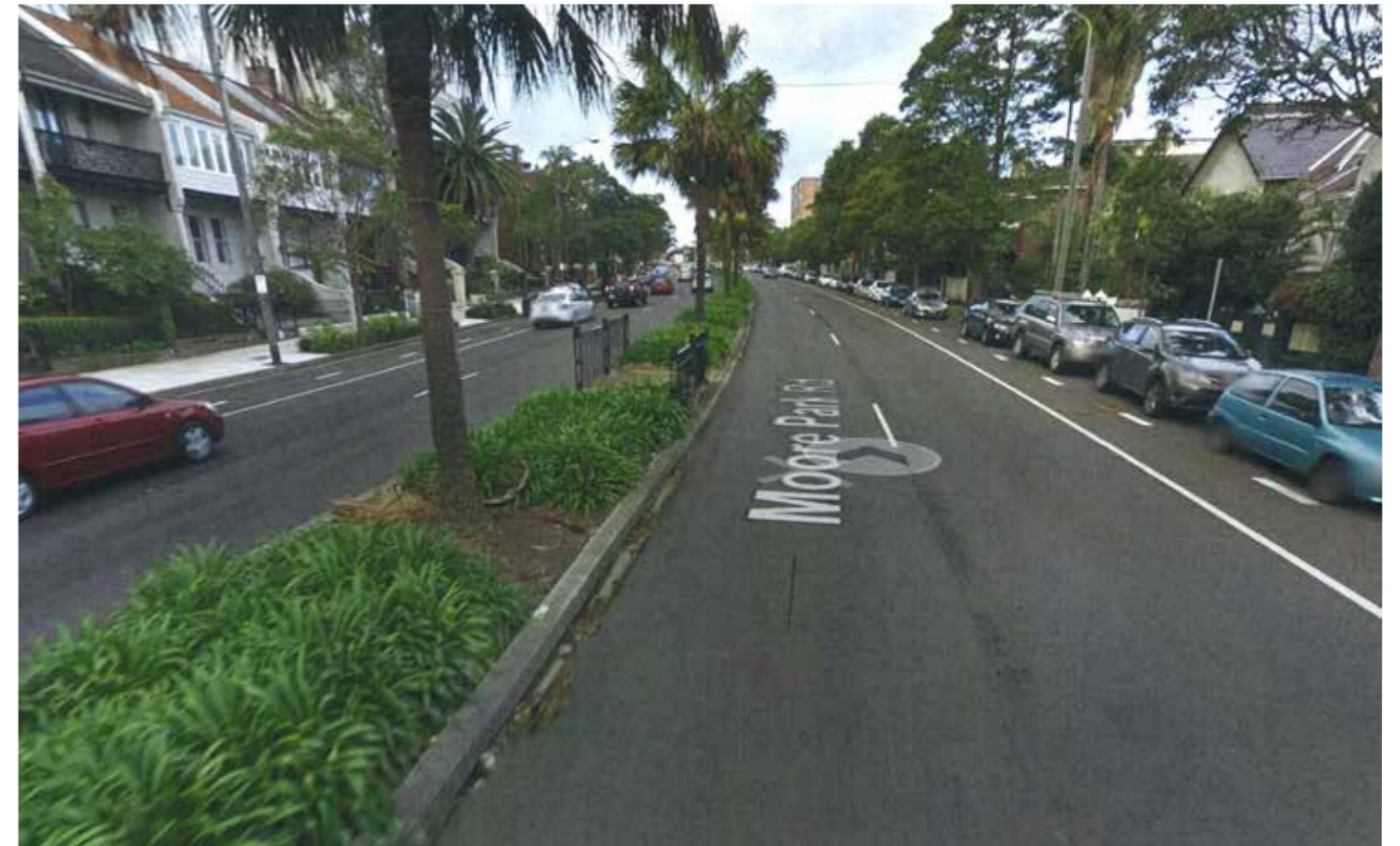
Example of an Escholts Kerb installed in Moore Park Road, Sydney
