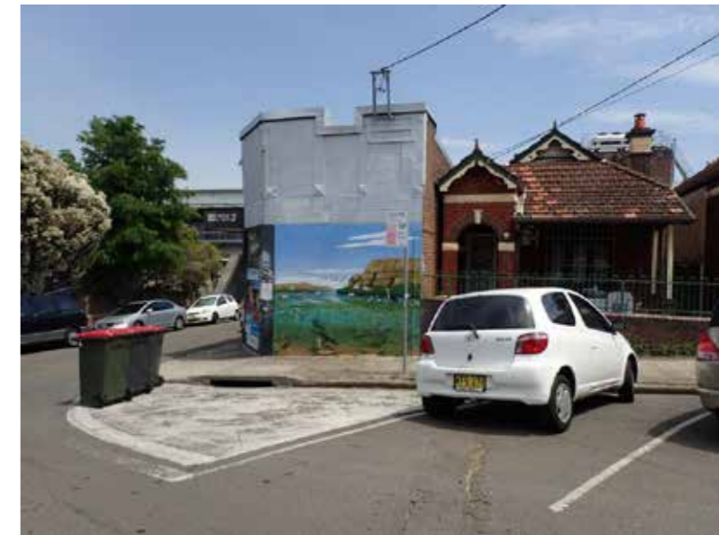
Two large areas of existing pavement have been used to define the parking bays and are designated as no parking areas in Wood St. These zones are currently painted areas on the pavement. These could be converted to raingardens to treat the stormwater runoff from the catchment.
