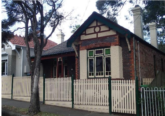
Figure 12: Dwellings east of the site in Tupper Street
