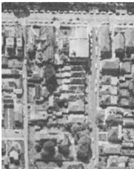
Figure 2.20 Detail of aerial photograph showing the Cyprus Club site in 1965. By this date Sparron had been demolished for the Newtown Rugby League Club clubhouse
