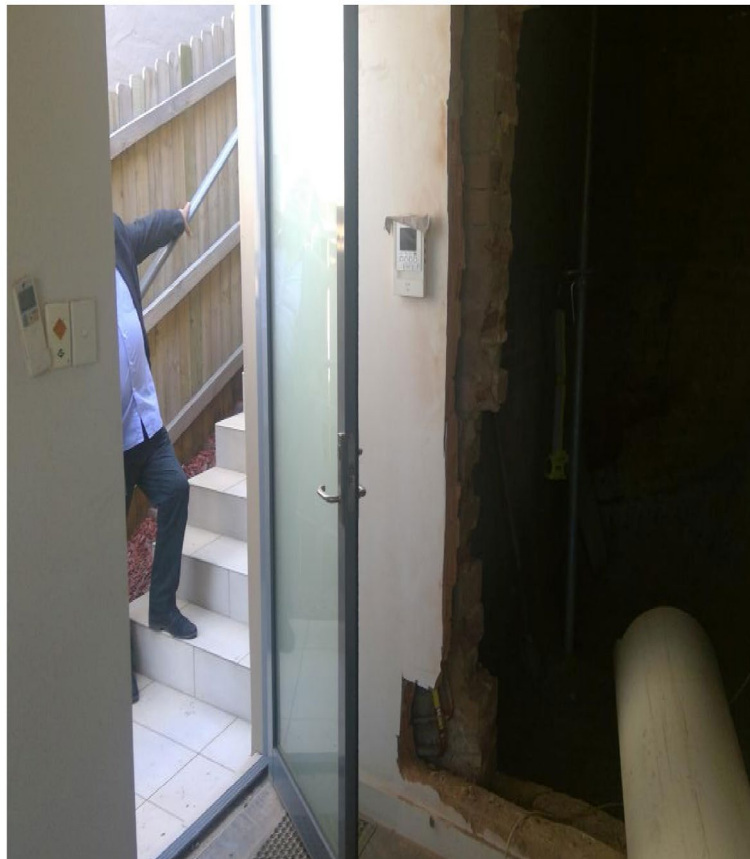
Figure 1 – Demolition works to rear wall of media room
