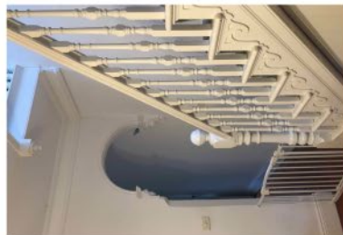
EXISTING STAIR - TO BE REBUILT AS COMPLYING STAIR TO THE BCA - NEWEL POST, BALUSTERS TO BE PRESERVED FOR REUSE
