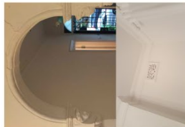
GROUND FLOOR EXISTING FRONT ROOM & ENTRY CORRIDOR - ALL ORIGINAL CEILING PLASTERWORK, ARCHWAY, DOORS, HARDWARE, SKIRTINGS & ARCHITRAVES TO REMAIN
