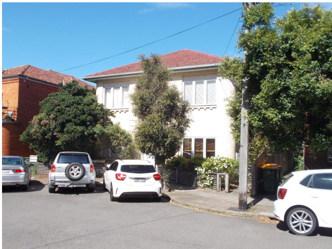
Picture 2 Site Photo – Allman Road Frontage
