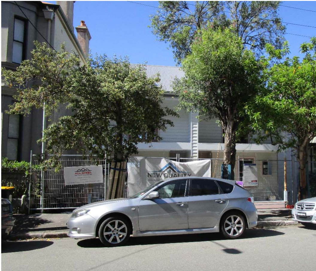
Figure 1: Dwellings currently under construction
