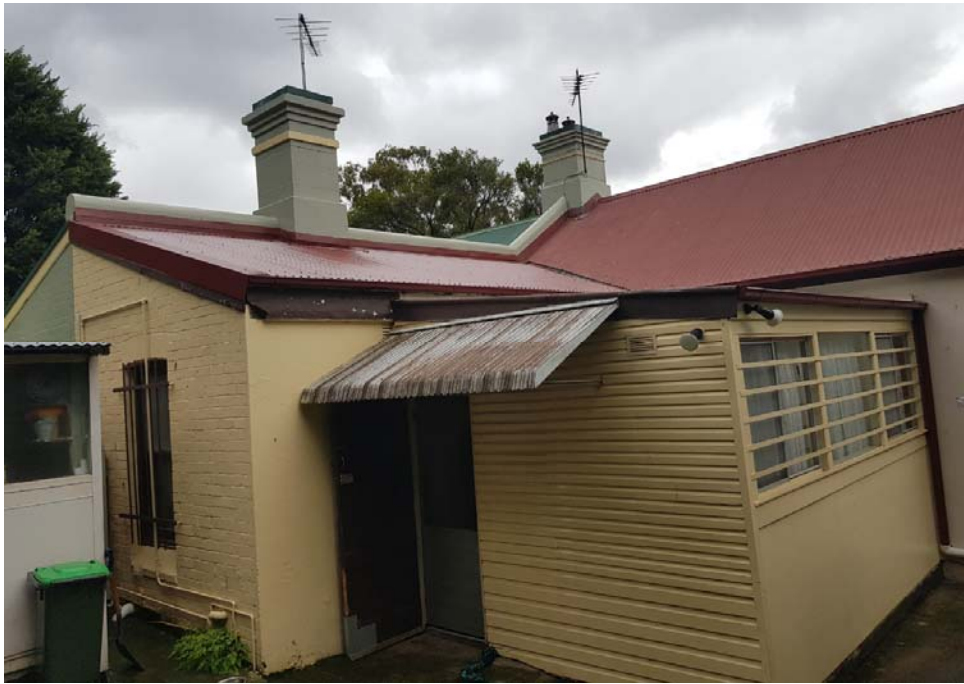
Image D. Rear of subject site.
