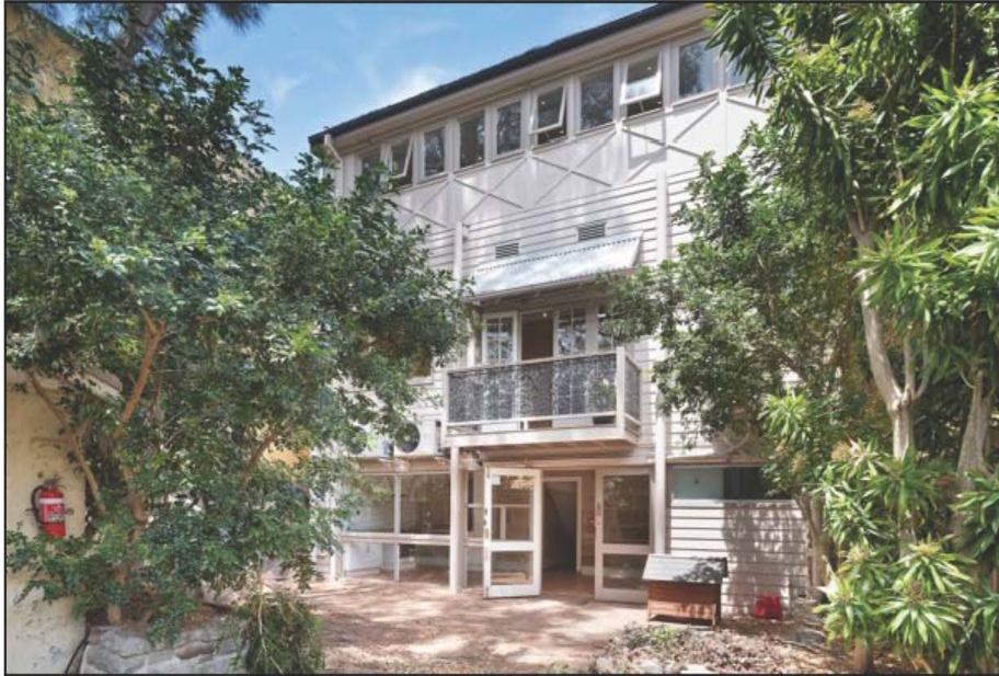
Photo 2 – View of rear of structure
