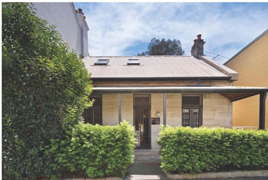
Photo 1- Building as viewed from Darling Street
