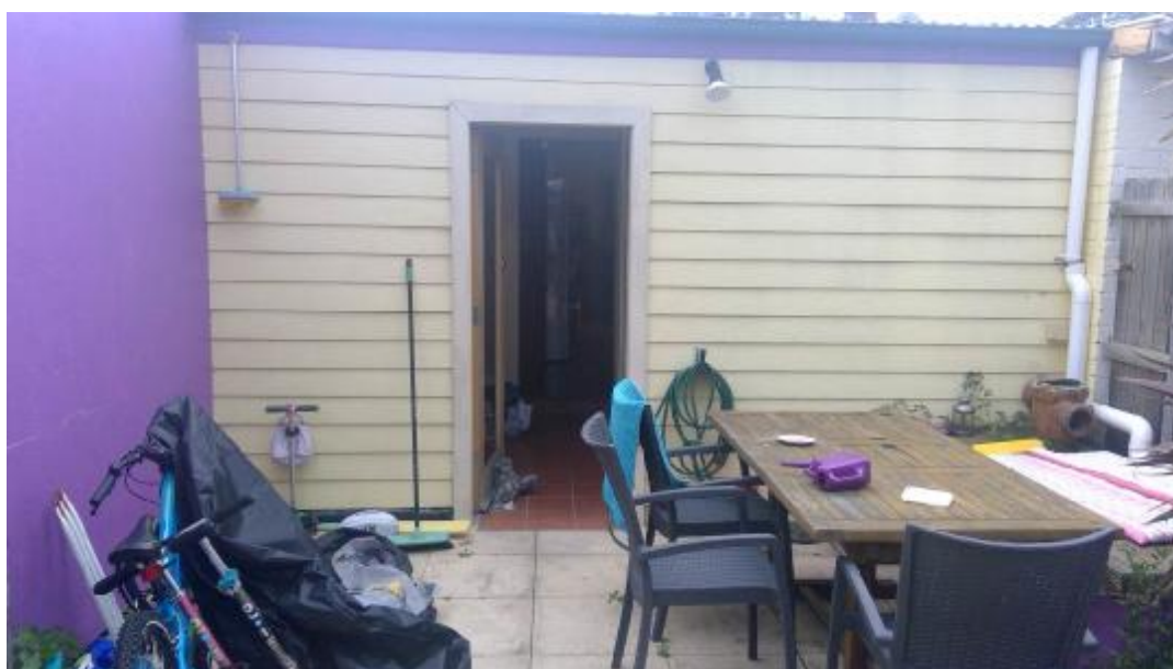
Figure 2 – Rear western wall of dwelling
