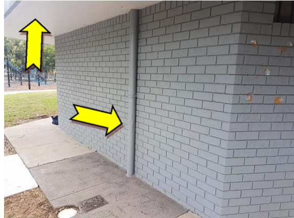
Photo 2. Exterior, walls and eaves – suspected lead-containing grey and white upper coloured paint systems.
