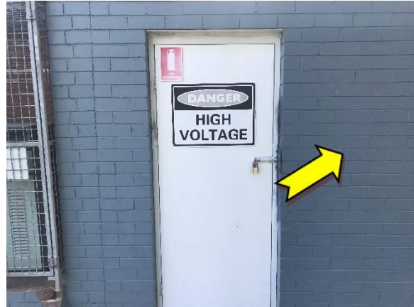
Photo 2. Exterior, throughout, wall – suspected lead-containing grey upper paint system.
