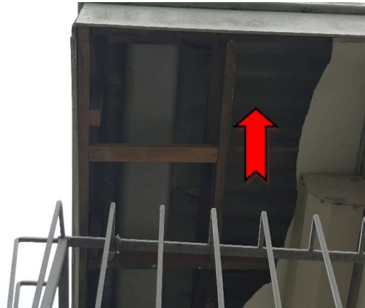
Photo 2. Exterior, throughout, roof – suspected asbestos-containing fibre cement sheeting.
