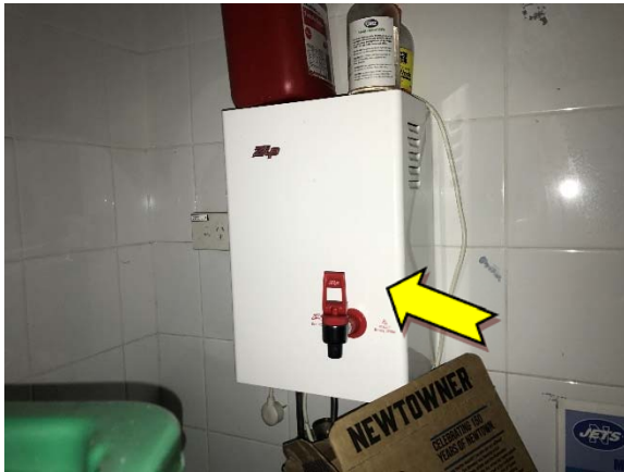
Photo 3. Interior, ground level, kiosk, hot water heater – suspected SMF internal insulation.
