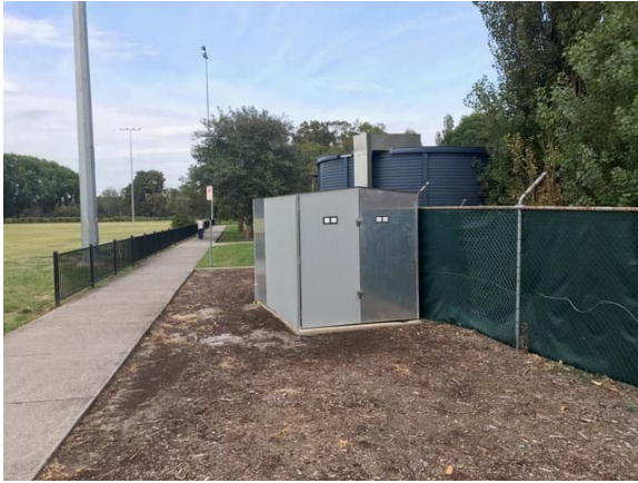
Photo 1. No hazardous materials identified or suspected at time of the Assessment.
