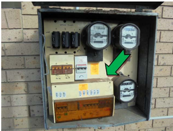
Photo 3. Exterior, southern wall, electrical backing board – non asbestos-containing fibre cement sheeting.
