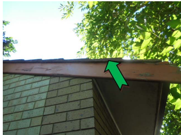
Photo 2. Exterior, throughout, under cloaking – non asbestos-containing fibre cement sheeting.
