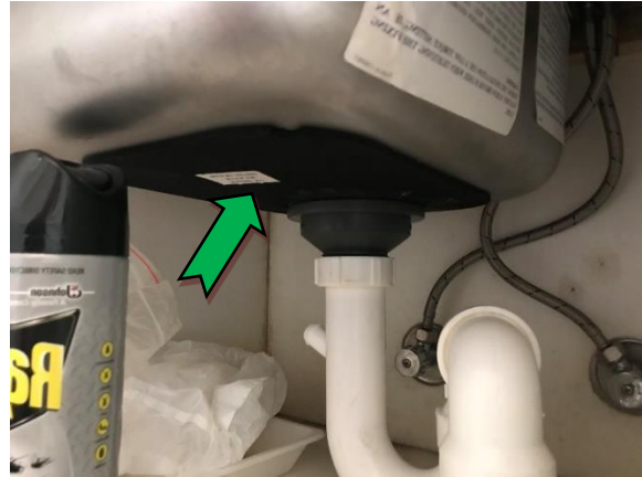
Photo 2. Interior, kitchen, under sink, sink pad – non asbestos-containing bituminous material.
