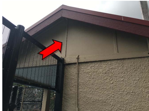
Photo 4. Exterior, ground level, eastern elevation, gable – asbestos-containing fibre cement sheeting.
