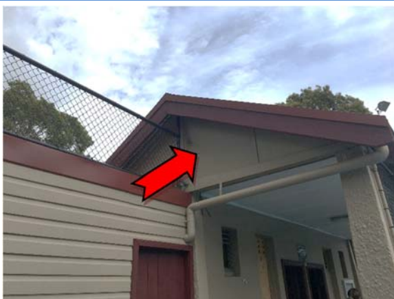
Photo 5. Exterior, ground level, western elevation, gable – assumed asbestos-containing fibre cement sheeting.
