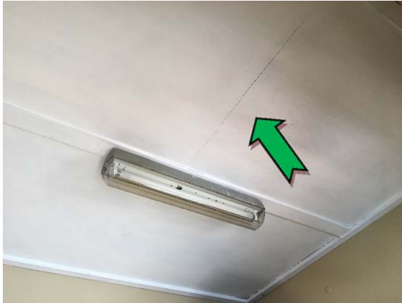
Photo 1. Interior, ground level, ceiling – non asbestos-containing fibre cement sheeting.
