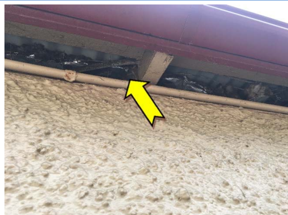
Photo 6. Interior, ground level – suspected SMF sarking insulation.
