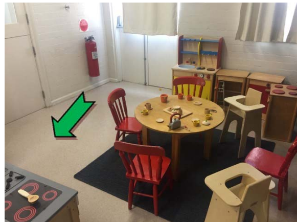
Photo 10. Interior, throughout, cream floor coverings – suspected non asbestos-containing sheet vinyl.
