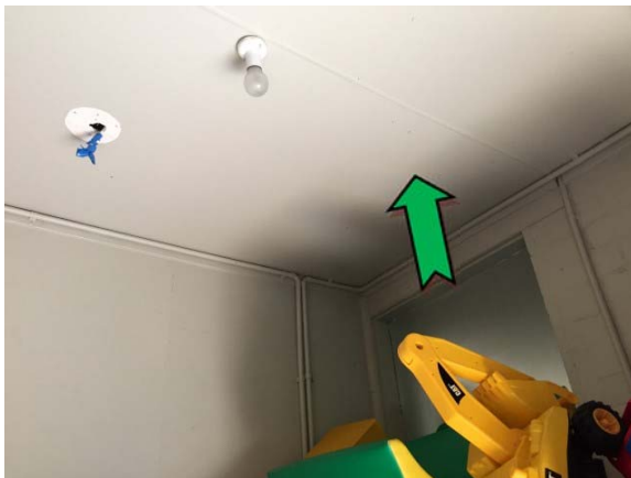
Photo 9. Interior, shed, ceiling – non asbestos-containing fibre cement sheeting.
