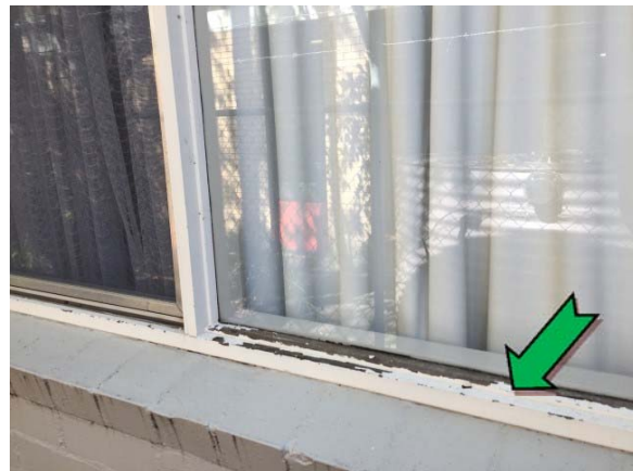
Photo 4. Exterior, southern elevation, window frames – non asbestos-containing window caulking.
