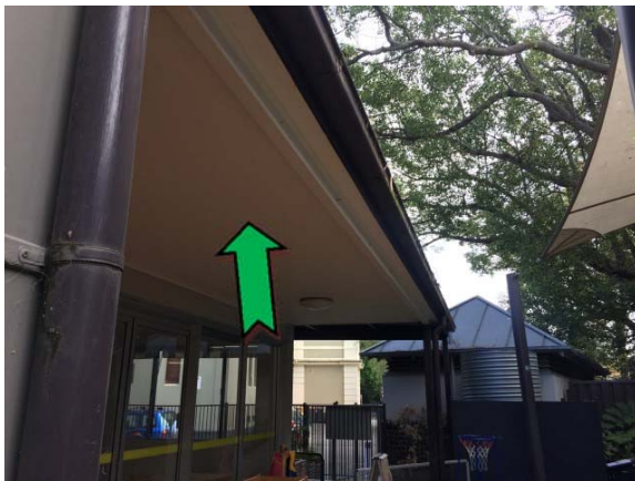
Photo 3. Exterior, awning – assumed non asbestos-containing fibre cement sheeting.
