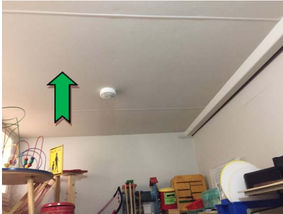
Photo 7. Interior, eastern store room, ceiling – non asbestos-containing fibre cement sheeting.
