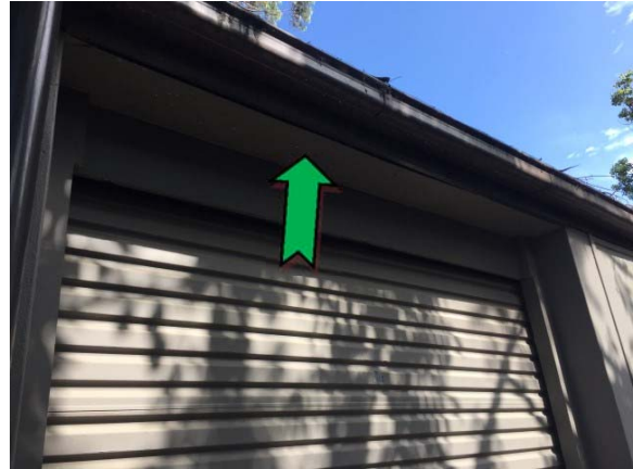
Photo 2. Exterior, eaves to shed – assumed non asbestos-containing fibre cement sheeting.
