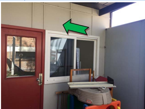
Photo 5. Exterior, southern elevation, wall – assumed non asbestos-containing fibre cement sheeting.
