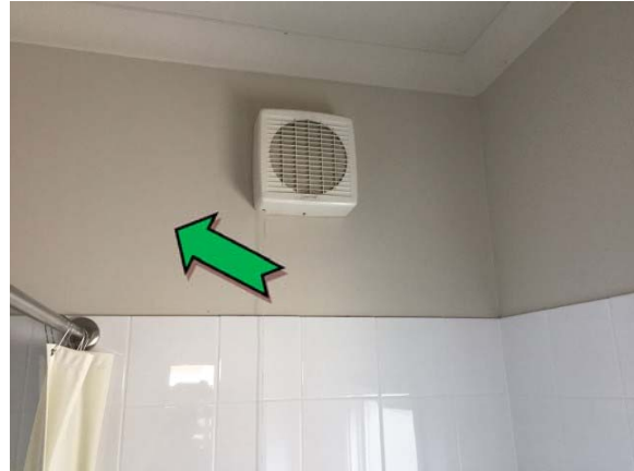
Photo 8. Interior, staff toilet, eastern elevation, wall – non asbestos-containing fibre cement sheeting.
