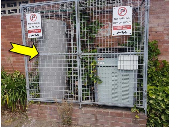
Photo 1. Exterior, north-east elevation, hot water heater – suspected SMF internal insulation.
