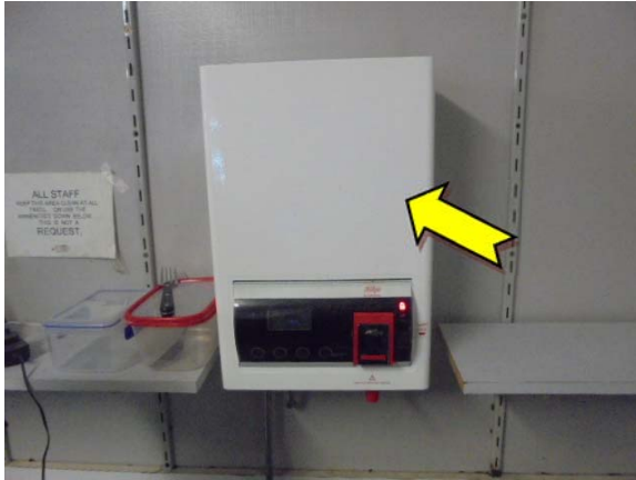
Photo Interior, ground level, kitchen, hot water heater – suspected SMF internal insulation. 1.
