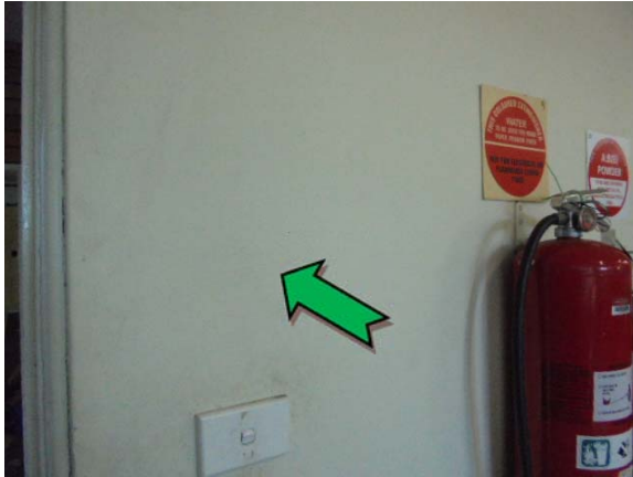
Photo 1. Interior, ground level, office and store room 1, walls – non asbestos-containing fibre cement sheeting.
