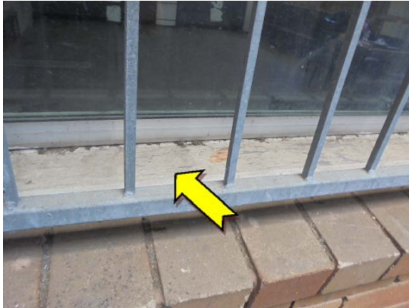
Photo 7. Exterior, throughout, window frames – suspected lead-containing cream upper paint system.
