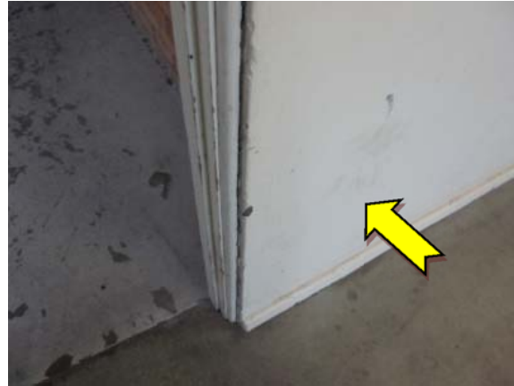
Photo 8. Interior, throughout, walls – suspected lead-containing white upper paint system.
