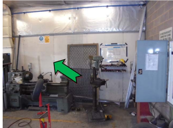
Photo 2. Interior, ground level, workshop, walls – non asbestos-containing fibre cement sheeting.
