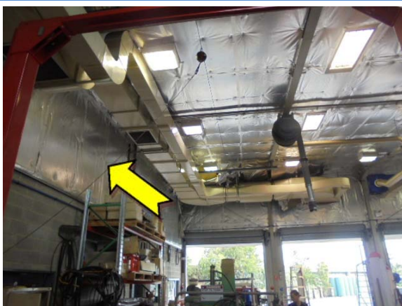
Photo 5. Interior, ground level, throughout ceiling and high level wall – suspected SMF sarking insulation.
