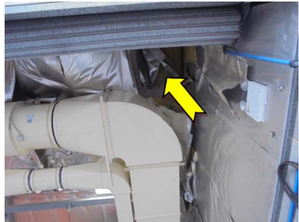
Photo 4. Interior, ground level, throughout, ceiling above SMF – suspected asbestos-containing fibre cement sheeting.
