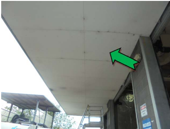
Photo 3. Exterior, north elevation, awning – non asbestos-containing fibre cement sheeting.
