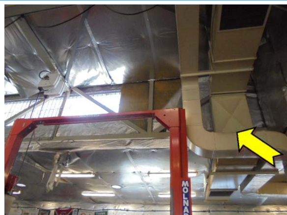
Photo 6. Interior, ground level, workshop, ductwork – suspected SMF internal insulation.
