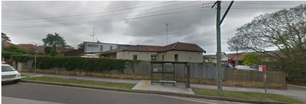
2 Bourne St side view
