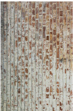
EXISTING BRICKWORK - STRIP PAINT - EXISTING WALLS
