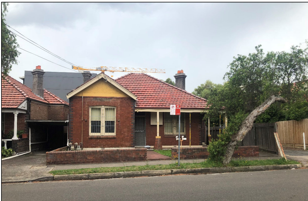
Image 1: Front of existing dwelling at No.59 Warren Road.
